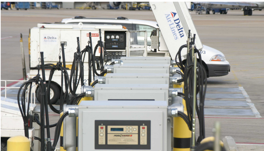
Two vehicles 'fill up' with electricity at one of the rapid recharge stations for electric vehicles at DFW airport.
